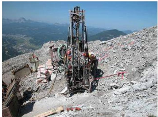
Figure 9. Air rotary drill used on South Peak during installation of subsurface geophones.
