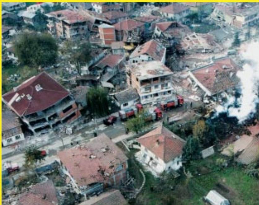
CRUMPLED BUILDINGS dot Düzce, Turkey, in the wake of a major tremor that struck in November 1999. Some scientists suspect that this disaster was triggered by an earlier shock near Izmit.
