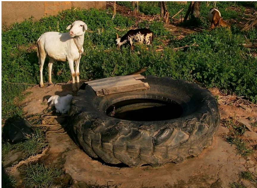
Figure C.2 Example of concrete and tire reinforcement (photograph by author)
