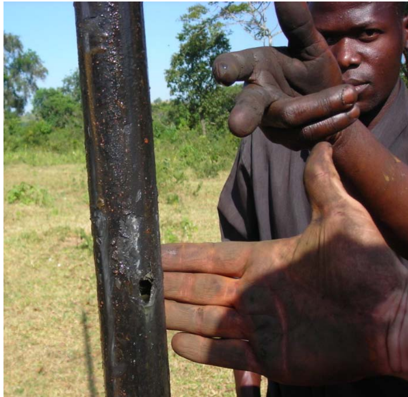
Figure 2.6 A hole eaten into an iron riser pipe from the Kyabasaija well (photograph by author)
